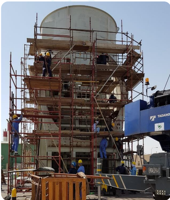
After Burner/Secondary Combusting Chamber fabrication
