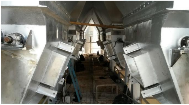
Erection of Hooper's
