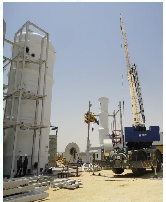
Scrubber Tank and Structure Assembly and Erection
