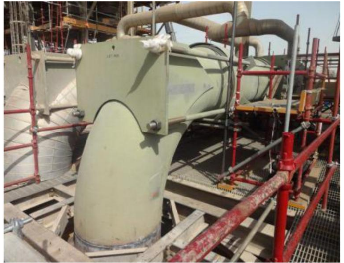
▲ Replacement of 42"Ø Air Line CS Pipeline Assembly along with the Expansion Joint Below. (4 th Floor)
