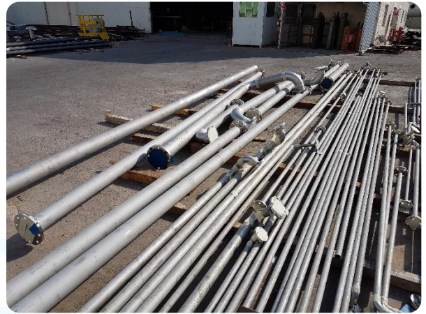
CS & SS Pipe fabrication completed
