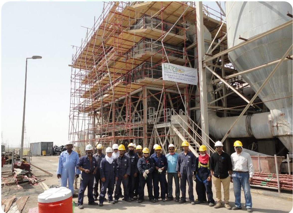
Replacement of Baghouse including electrical & Instrumentation
