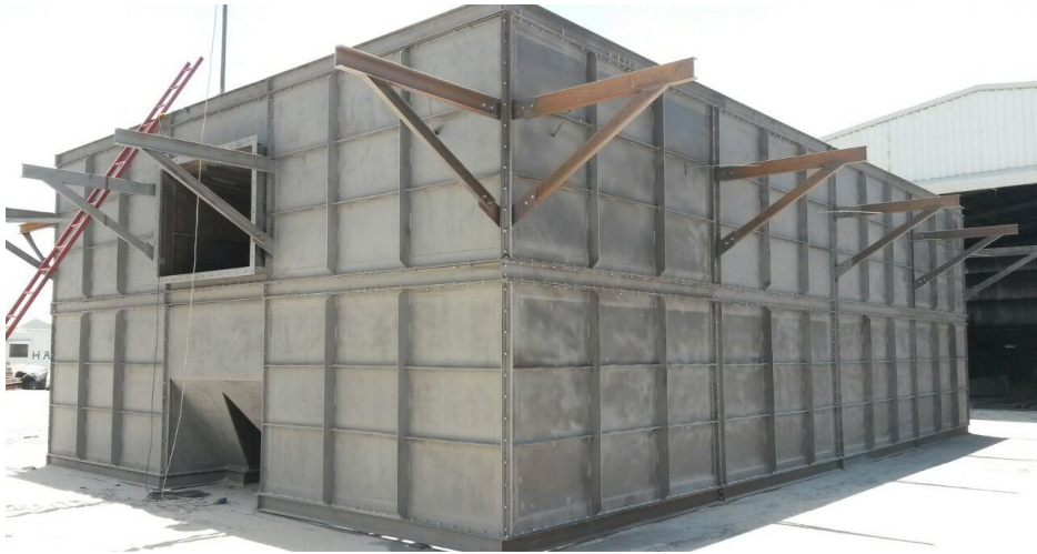
Fabrication of Baghouse Panels
