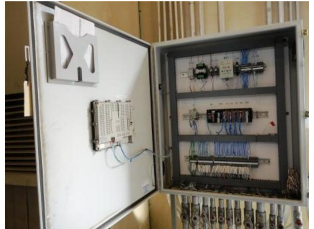
▲ Installation of Annunciator Panel Board
