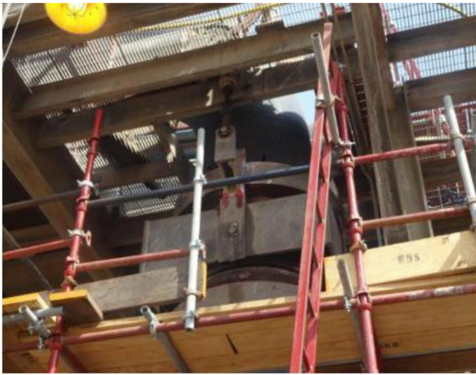
▲ Replacement of Expansion Below Gimbaled Joint 42"Ø HC Line SS Pipeline. (4 th Floor)
