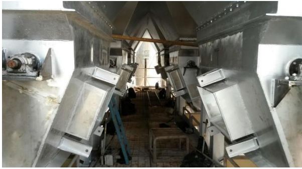
Erection of Hooper's
