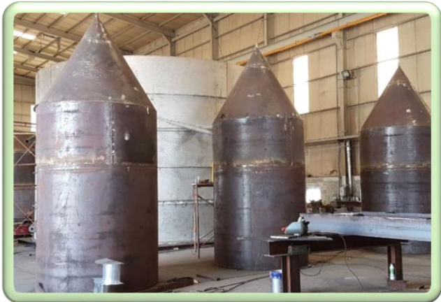
FGE & AW TANKS
