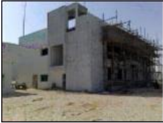
Euro Gulf Admin Building (While under construction)
