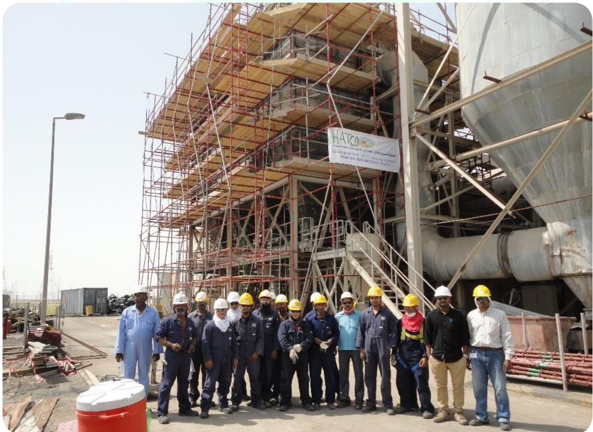
Replacement of Baghouse including electrical & Instrumentation
