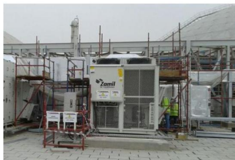
Aromatics MCC Building in SADARA Complex.
