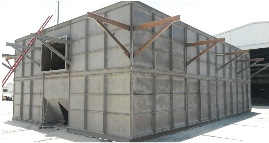
Fabrication of Baghouse Panels
