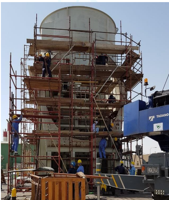
After Burner/Secondary Combusting Chamber fabrication
