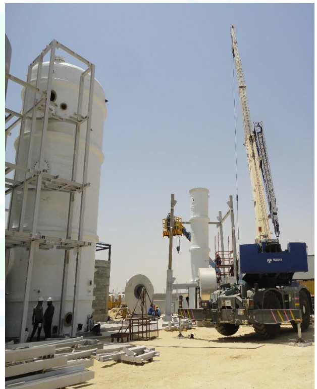
Scrubber Tank and Structure Assembly and Erection
