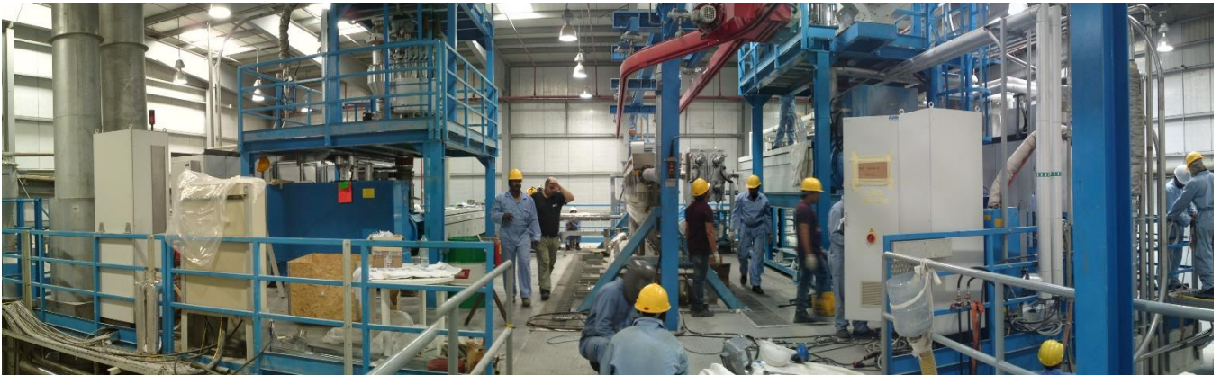
Erection of Equipment's and Structural Steel that will serve as platform for the new machines
