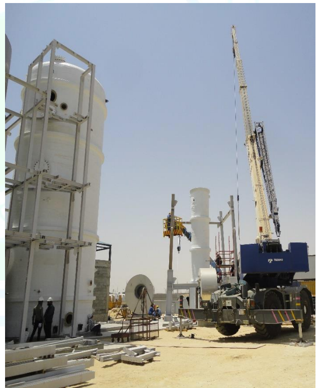
Scrubber Tank and Structure Assembly and Erection
