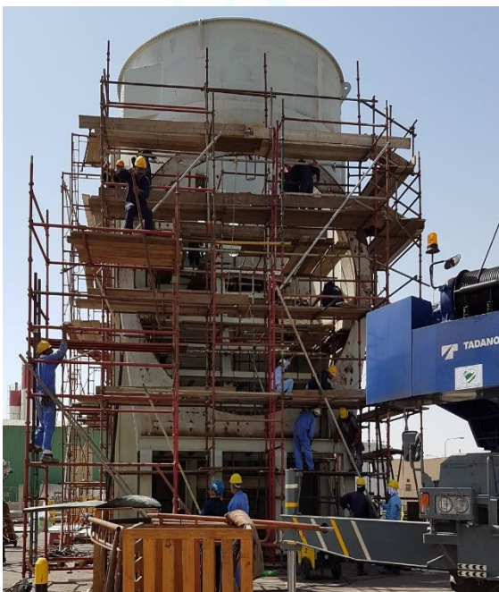
After Burner/Secondary Combusting Chamber fabrication
