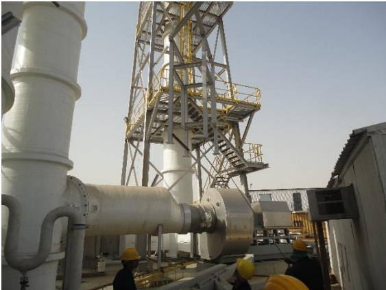
Scrubber to Stack Assembly
